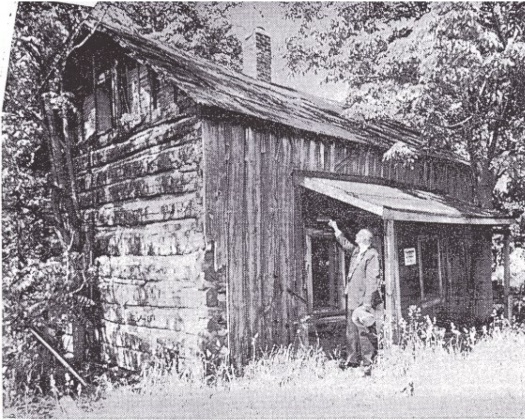
Last log cabin is checked over by the county historian, W. Glenn Norris. The cabin on Conlin Rd. in North Lansing went unnoticed for a long time because of sheathing which covered the original logs. (Ithaca Journal, 17 June 1958)
